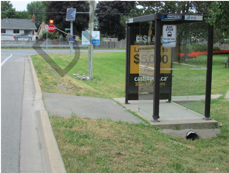
Figure 7: A non-accessible stop which lacks a physical barrier between the deployment area and a steep slope.
