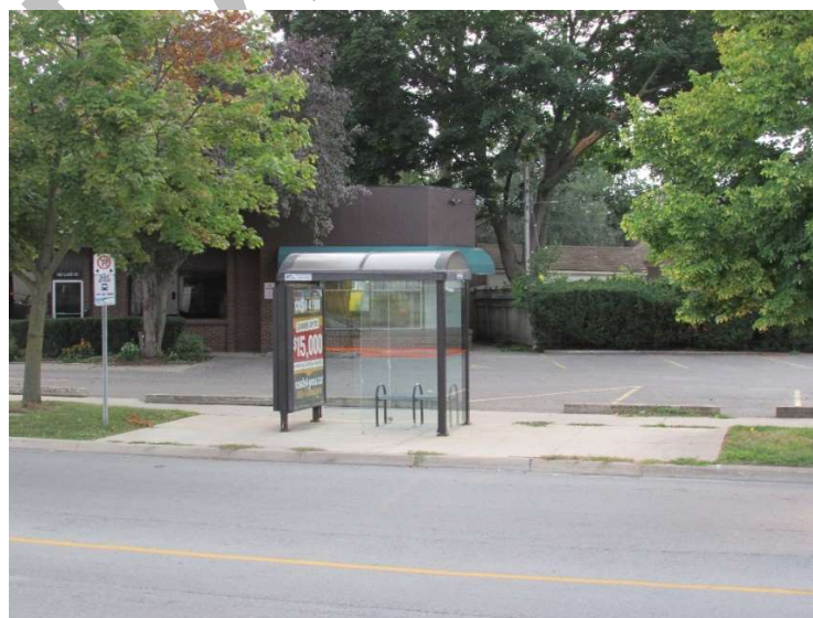
Figure 6: A stop with smooth unobstructed surfaces between the loading area, sidewalk and passenger amenities.
