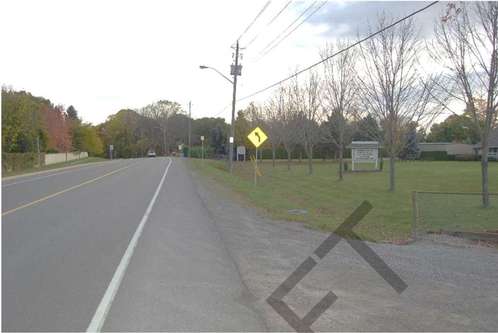
Figure 3: Non-accessible bus stop on a rural road with no landing pad or sidewalk.
