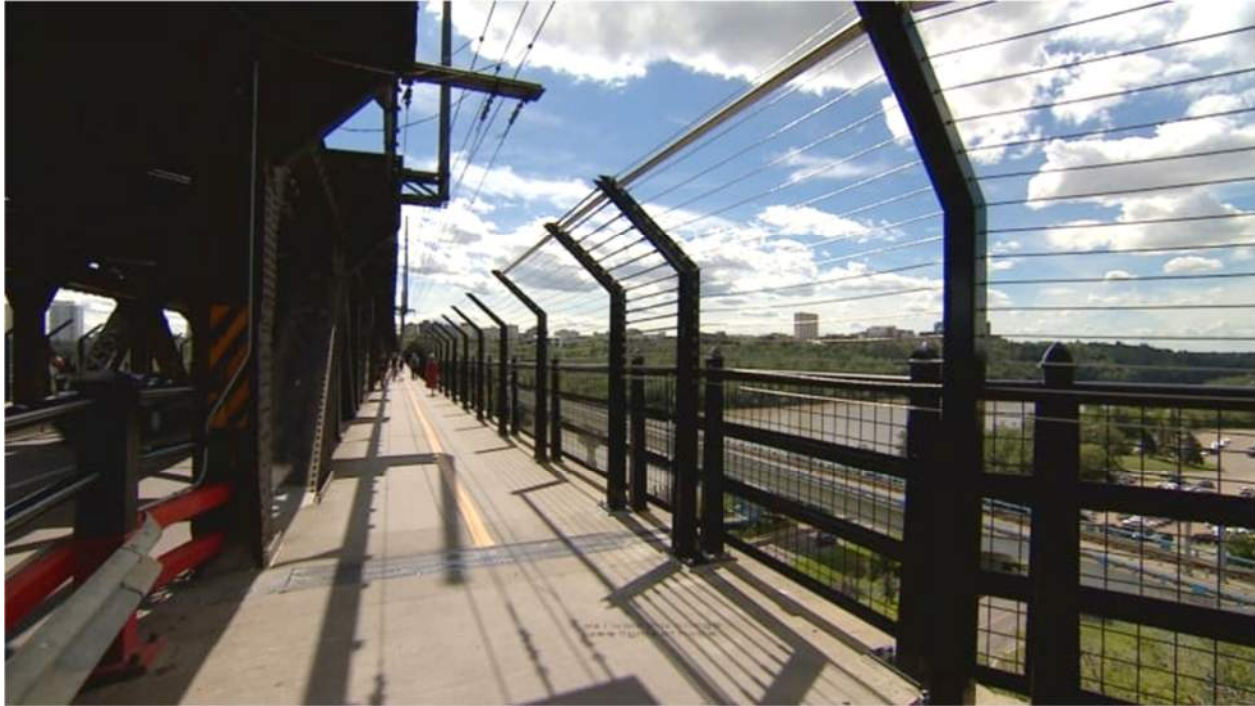
Figure 2.6 – High Level Bridge Barrier (Suicide, 2017)
