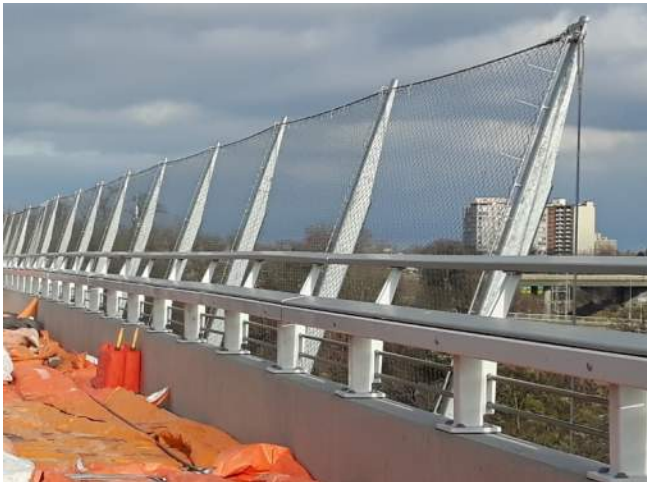
Figure 1.3 – Existing Debris Barrier
