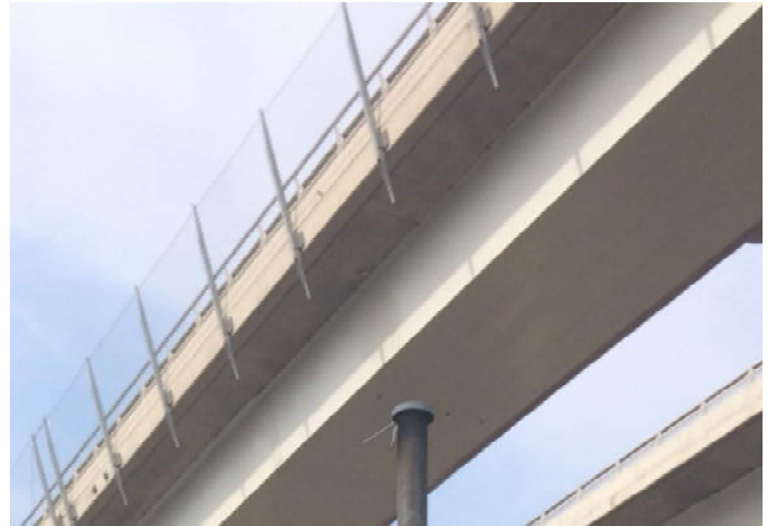
Figure 1.3 – Existing Debris Barrier
