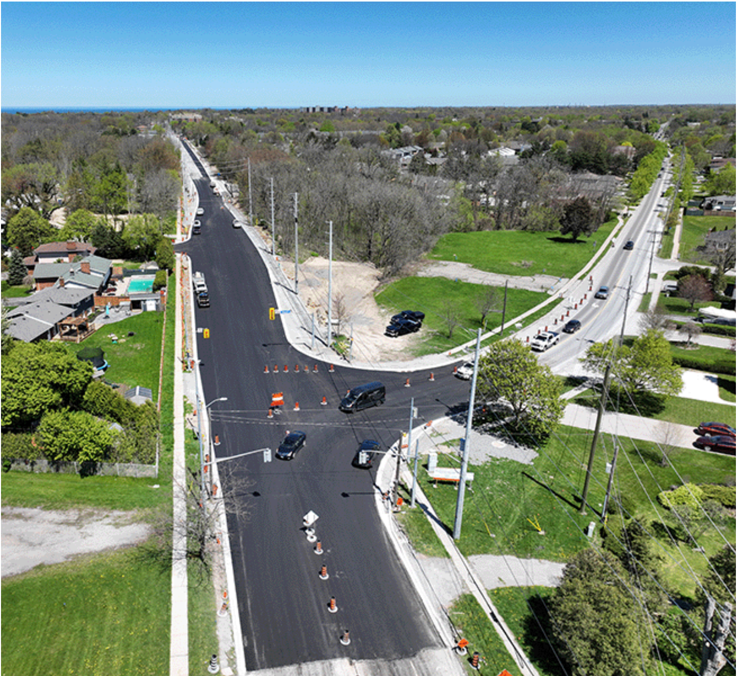
Intersection Reconstruction Ontario Street (RR 42)
