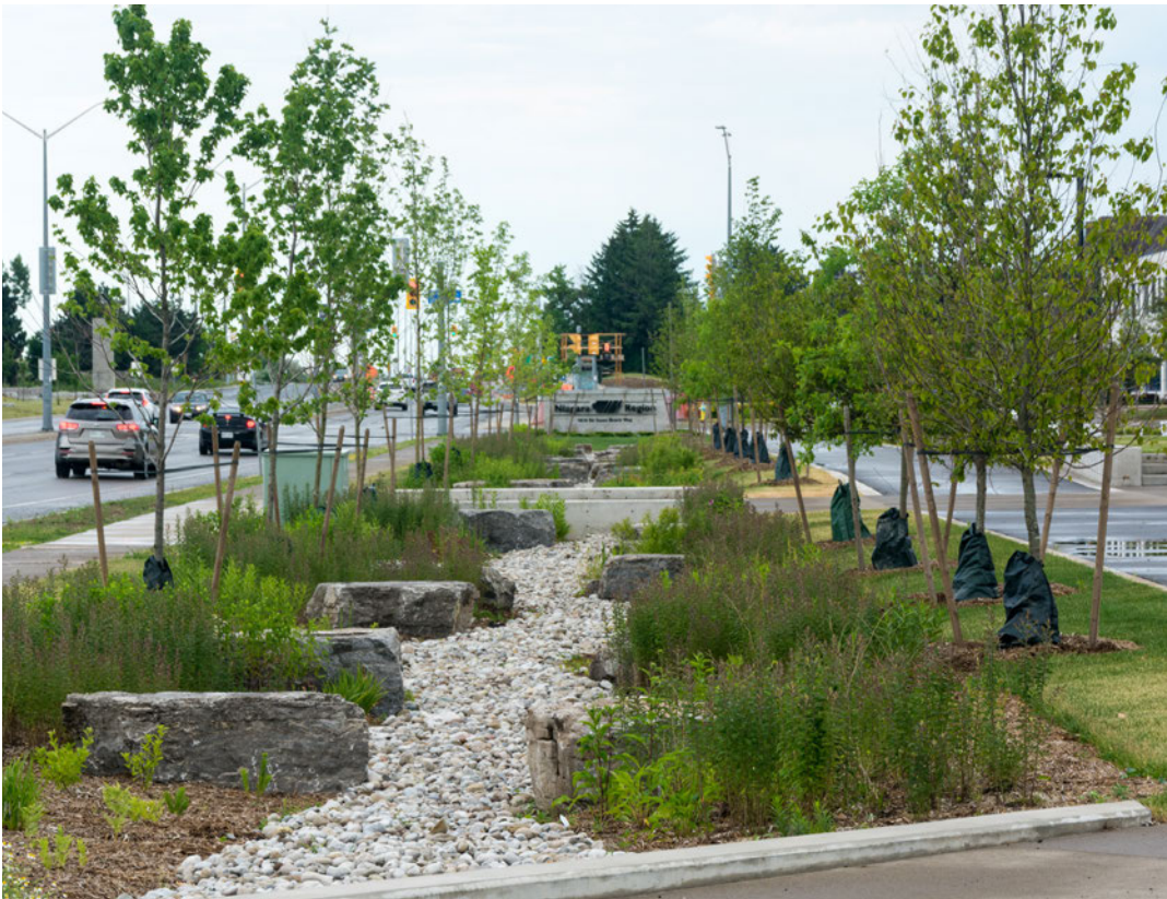
Figure 13: Bioswales located at walkways and parking lots can collect stormwater runoff to minimize the dependency on stormwater sewers.
