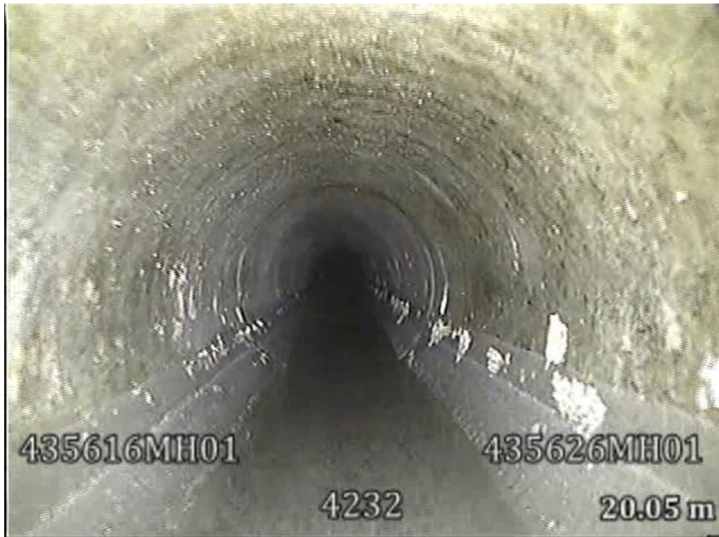
Picture 1: Huron Street Sewer after Cleaning – mid 2018
