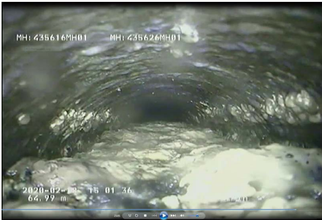
Picture 2: Huron Street Sewer - February 2020
