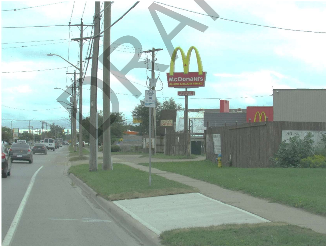
Figure 4: Landing pad is long and deep enough to deploy the ramps and have space to manoeuvre.
