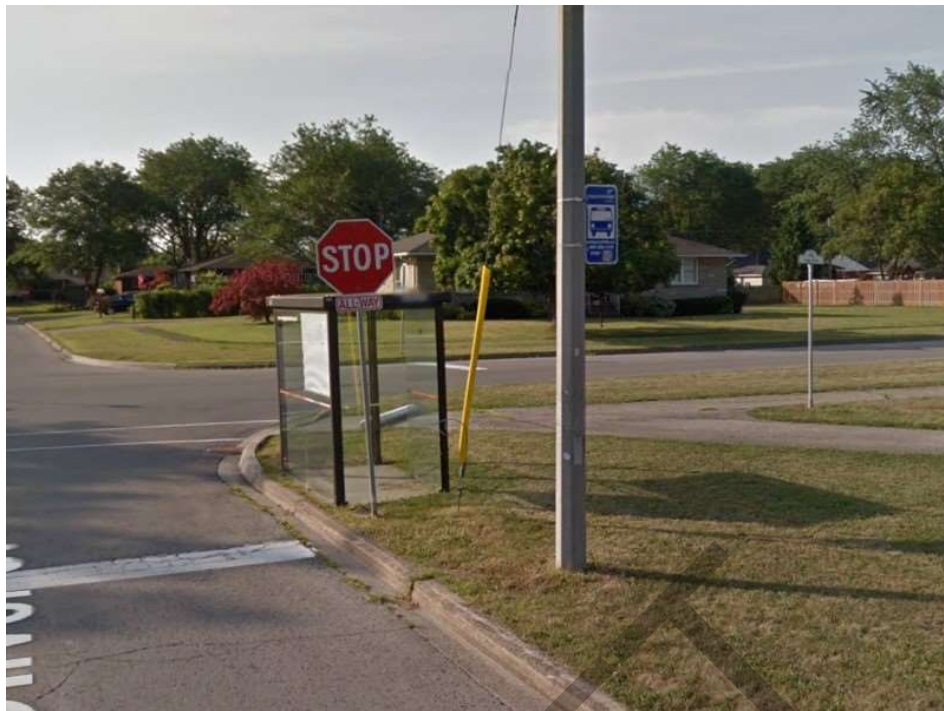
Figure 9: A non-accessible bus stop with a utility guide wire obstructing the landing area with reflective sheath.
