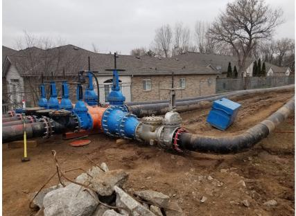
Complex bypass piping systems are installed to carry the flows from the bypass pumps to a discharge point downstream of the project site approximately two (2) kilometers away.
