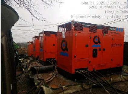
Complex bypass systems are installed upstream of the project to divert the sewage around the project site. CIPP Installations require dry working conditions.
