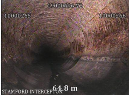
Hydrogen Sulfide gases have deteriorated the concrete in the sewer thus exposing and attacking the rebar reinforcement.
