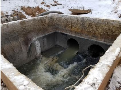
Hydrogen Sulfide gases have deteriorated the concrete in the manhole above sewage levels thus exposing and attacking the rebar reinforcement.
