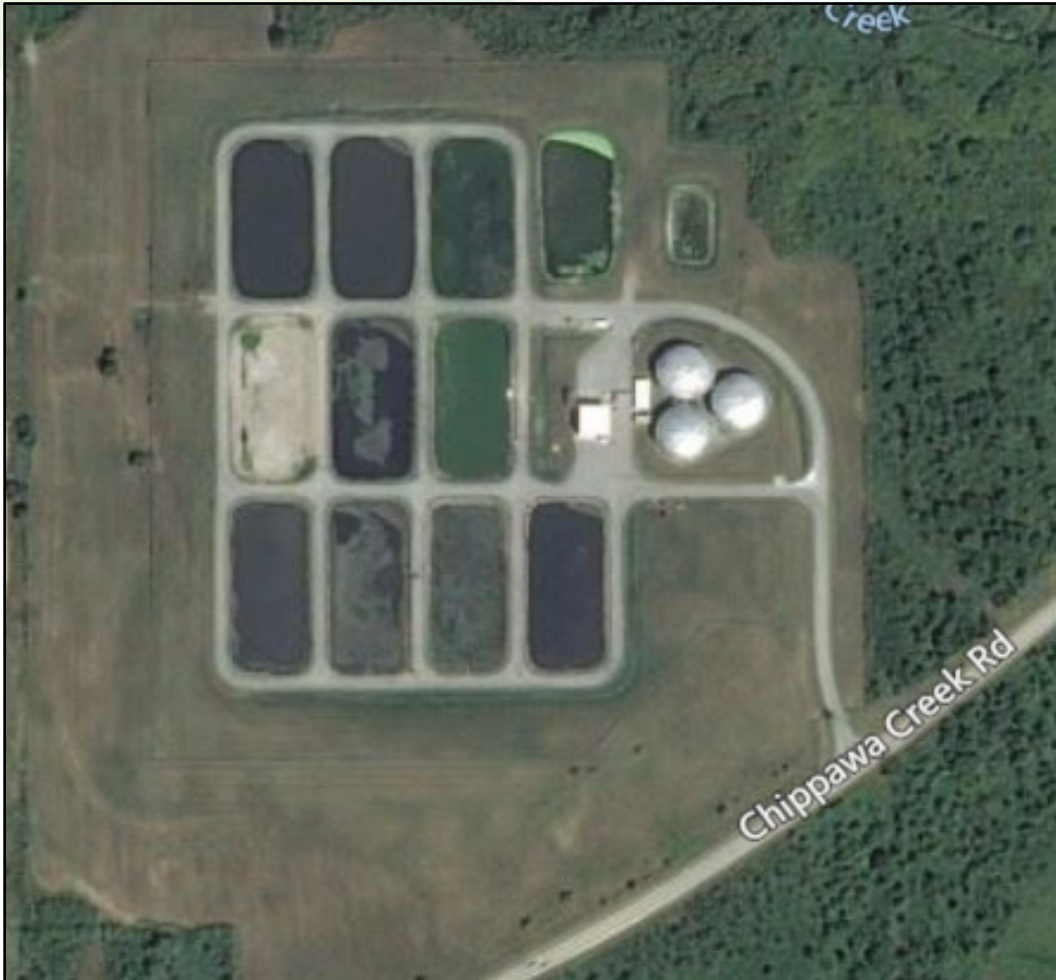
Garner Road Biosolids Facility
