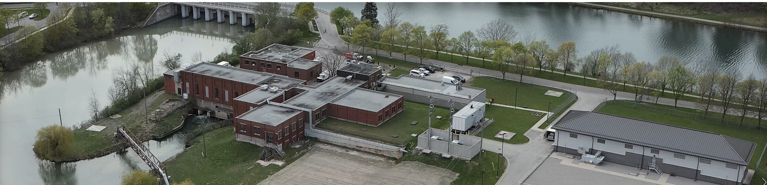
Welland Water Treatment Plant
