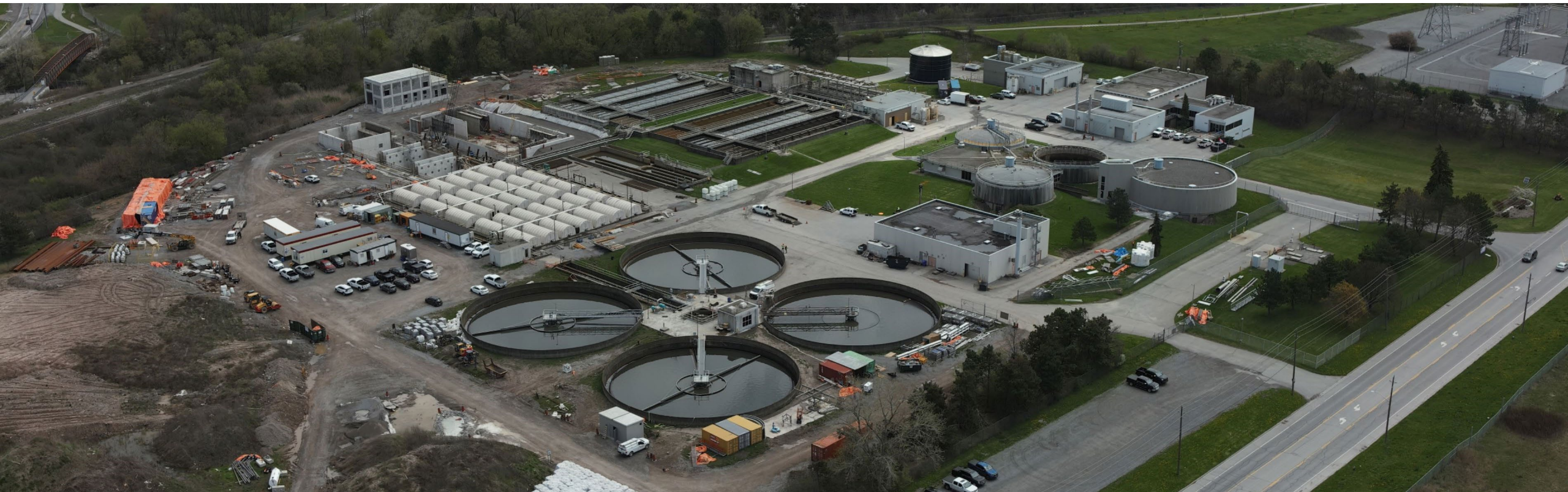
Niagara Falls Wastewater Treatment Plant
