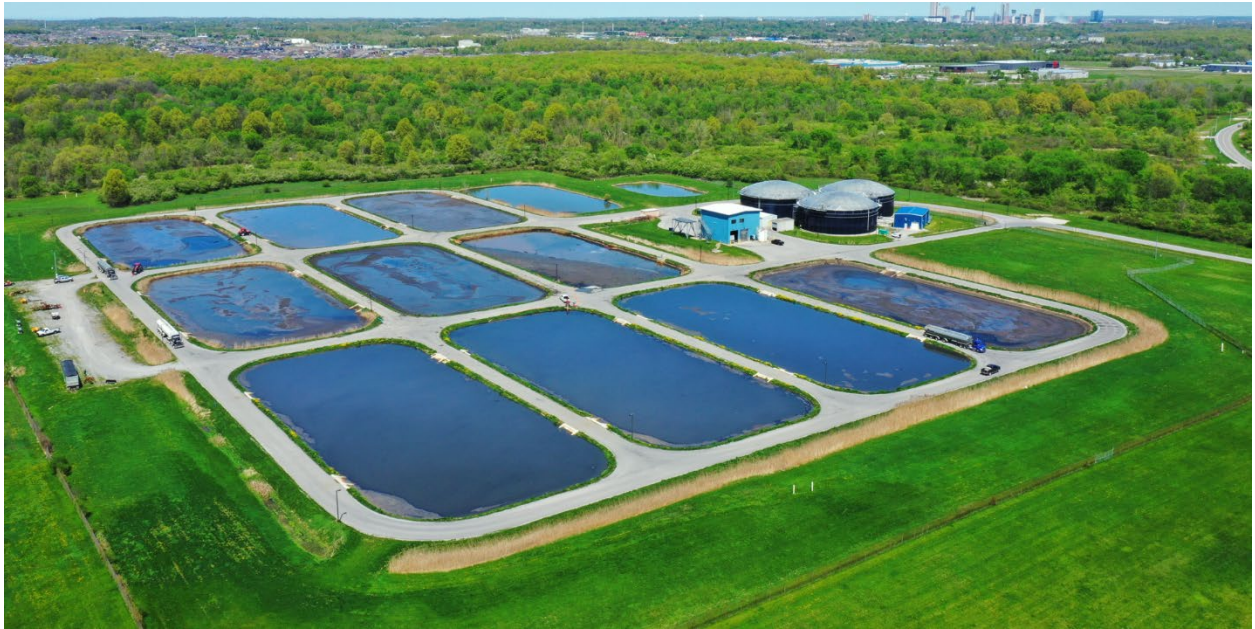
Figure 1-Garner Road Biosolids Facility Aerial View showing the 10 lagoons.
