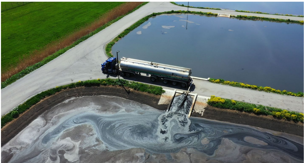
Figure 4-Picture of Transfer of Trucked Liquid Biosolids Material to a storage lagoon.
