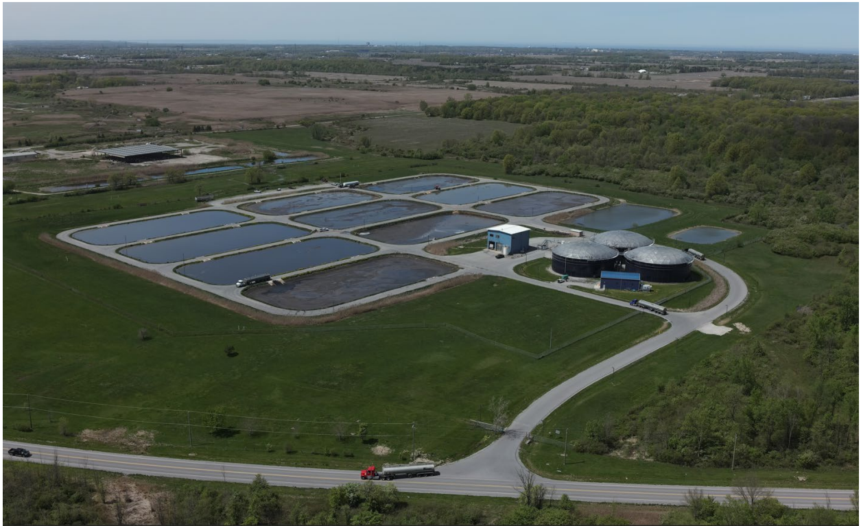
Figure 2-Garner Road Facility - Facing North
