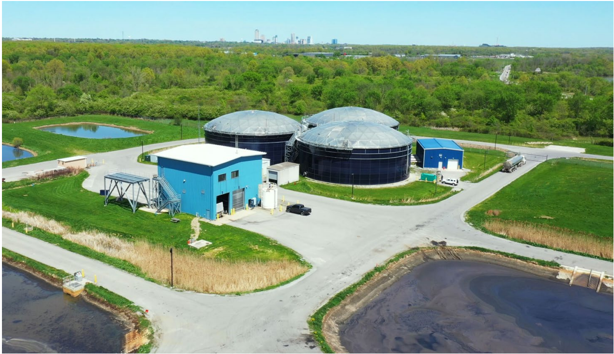
Figure 3-Garner Road Centrifuge Building and Circular Storage Tanks
