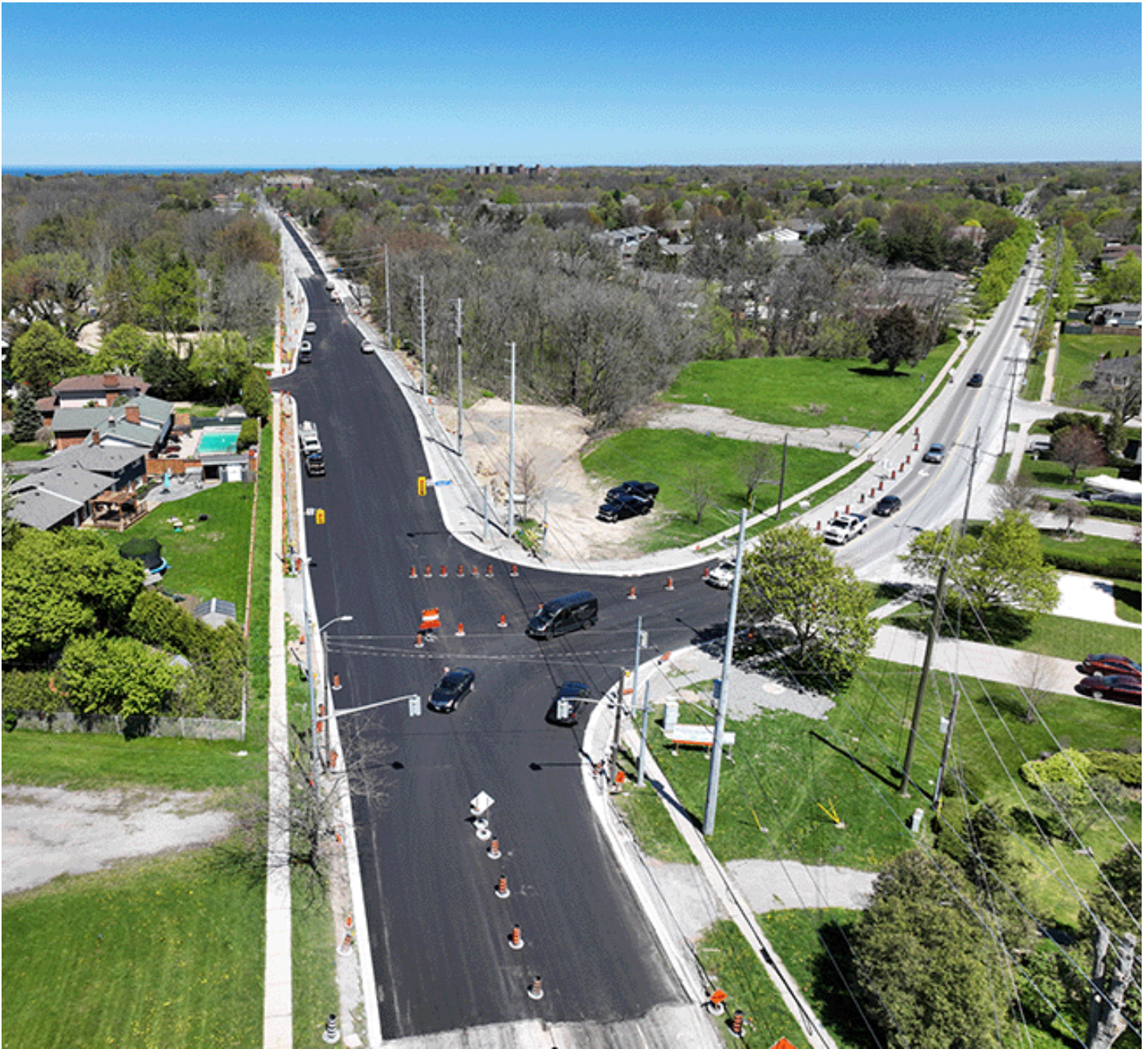
Intersection Reconstruction Ontario Street (RR 42)
