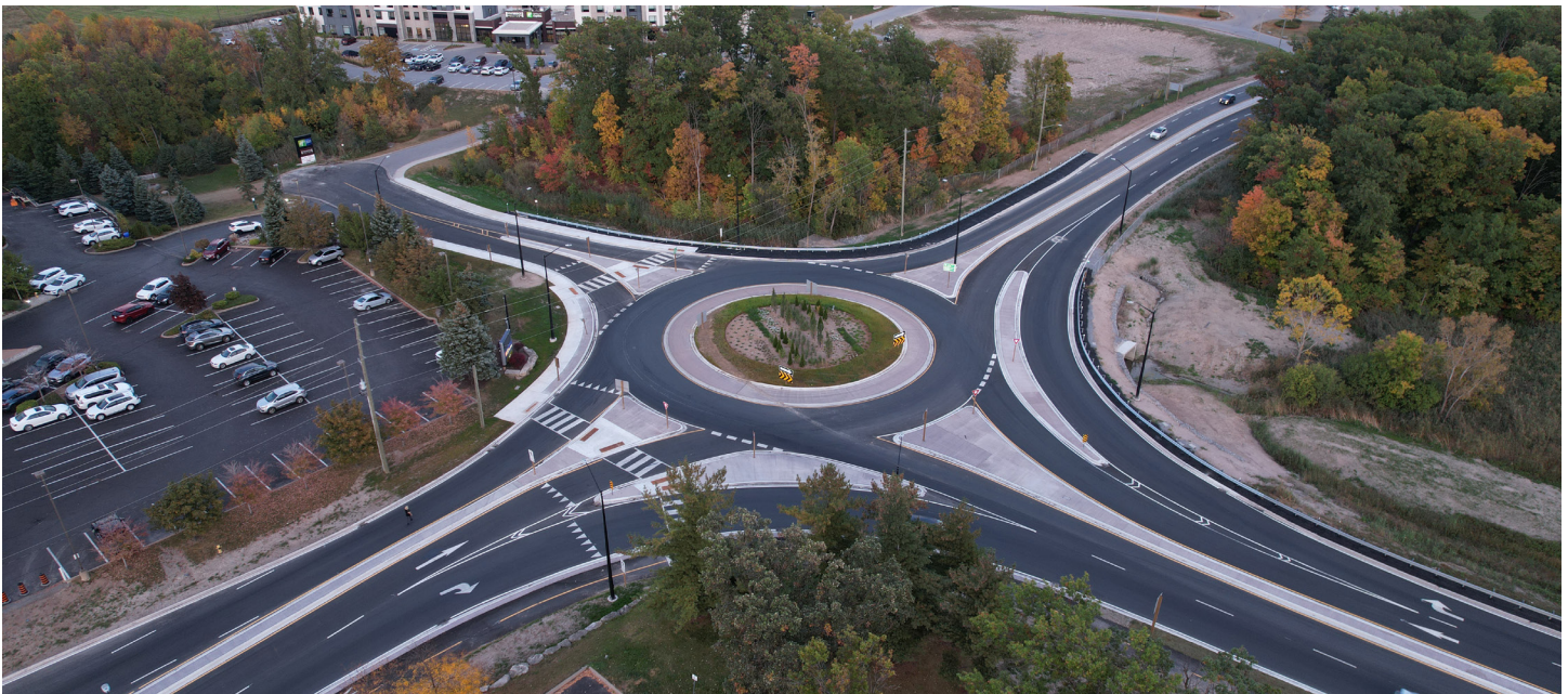
Roundabout: York Road (RR 81) at Glendale Avenue (RR 89)
