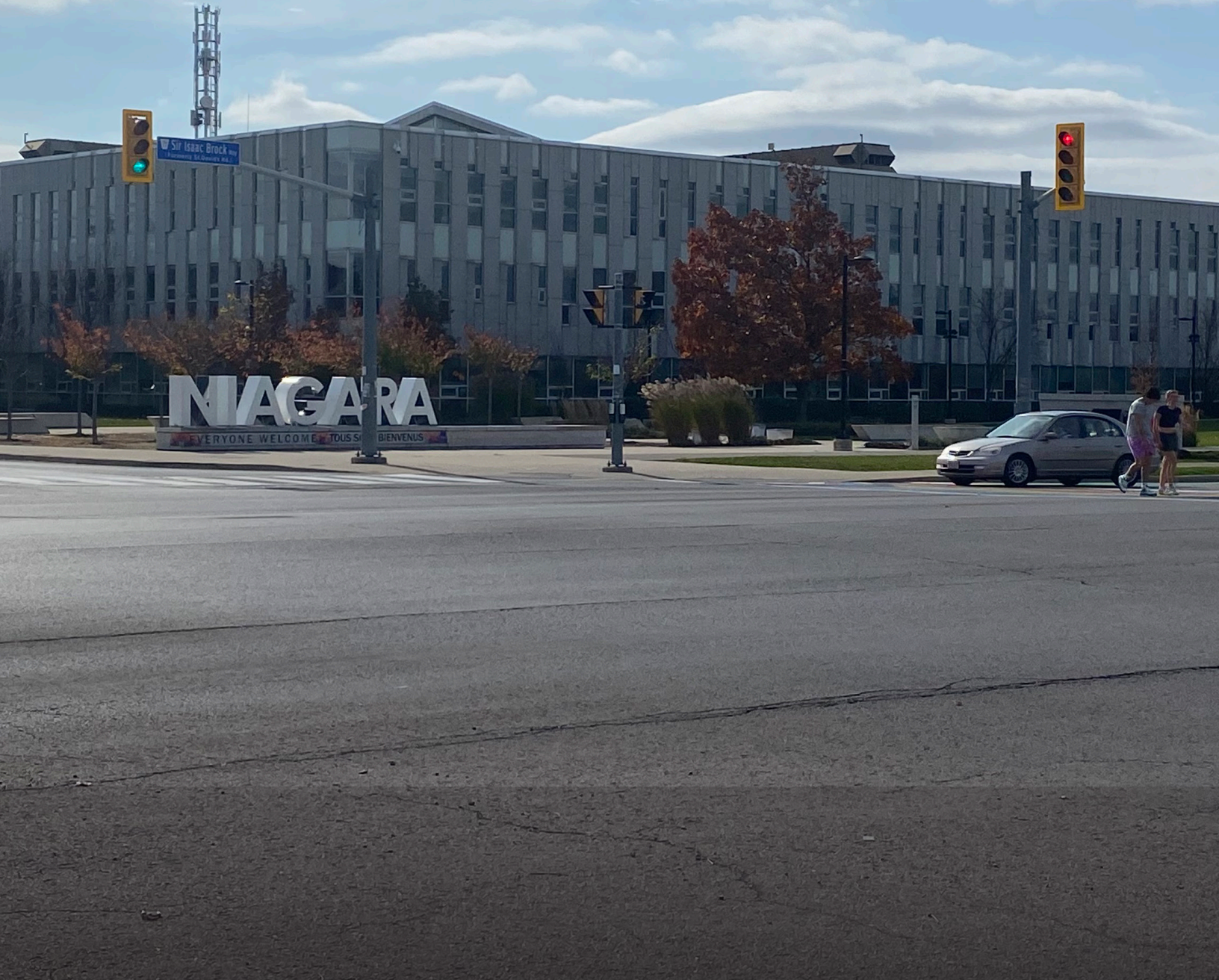
Niagara Regional Headquarters at Sir Isaac Brock Way and Schmon Parkway
