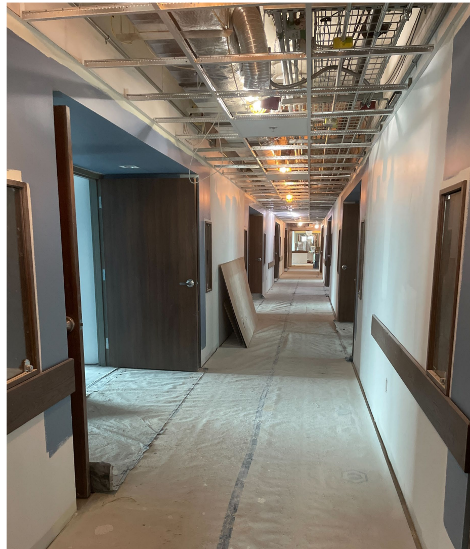
Resident Home Area Corridor
