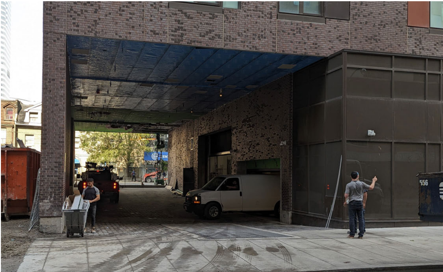
Figure 142: Waste collection areas should have an overhead clearance of 4.4 metres to ensure collection vehicle access is achievable.
