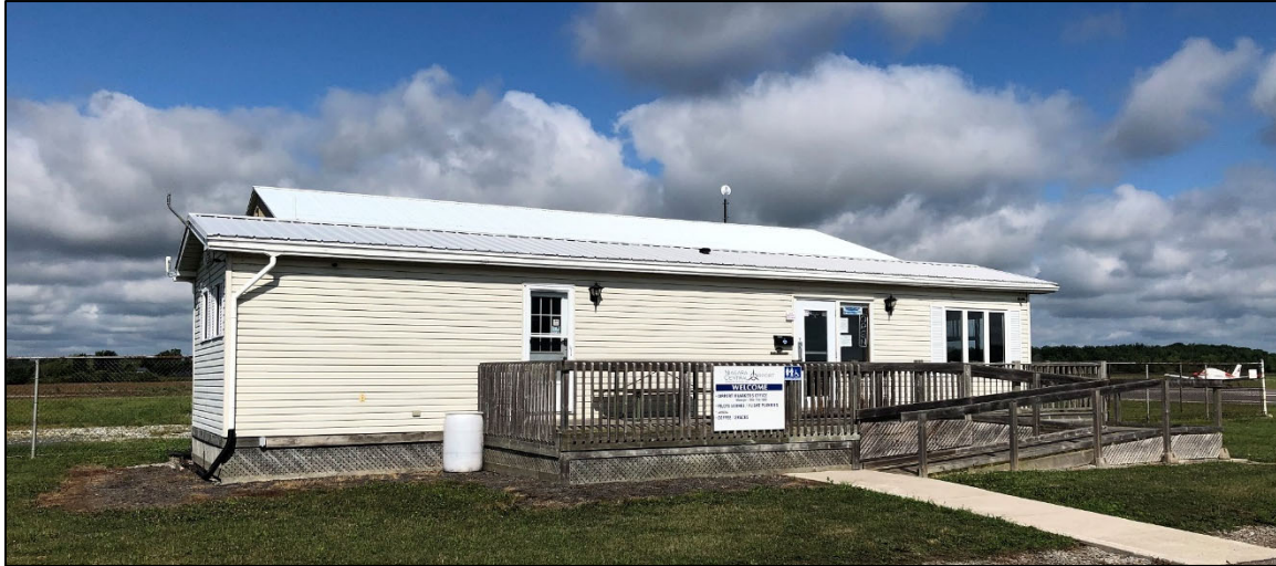
Terminal Operations Building at Niagara Central Airport
