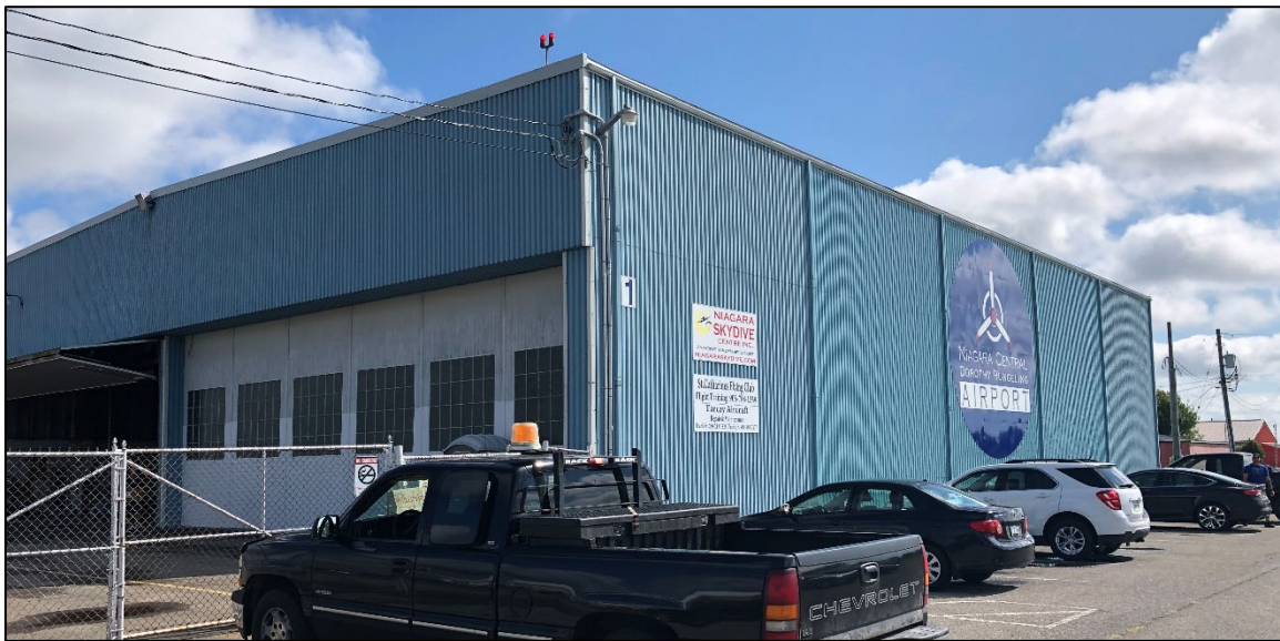
Hangar 1 at Niagara Central Airport
