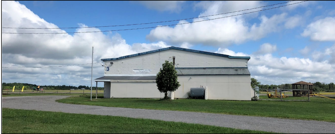
Hangar 3 at Niagara Central Airport
