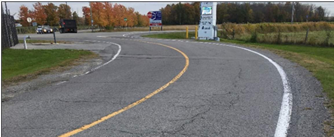
Main Access Road at Niagara District Airport
