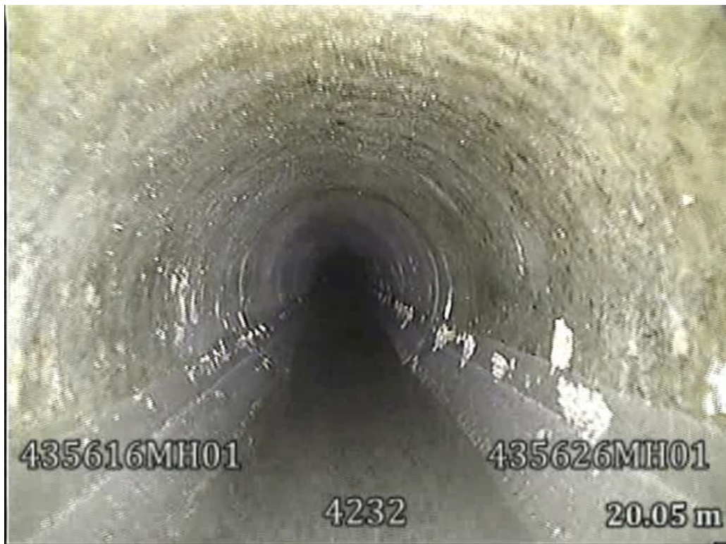
Picture 1: Huron Street Sewer after Cleaning – mid 2018
